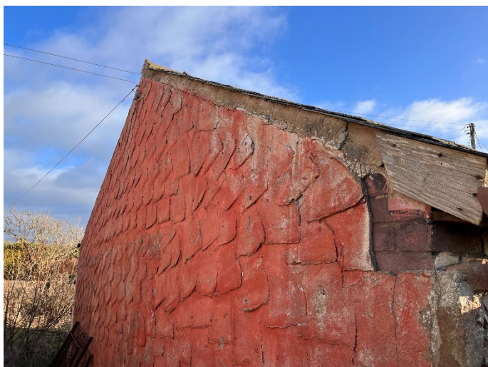
Well sealed walls
